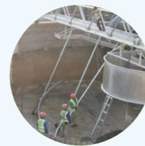
Renovation of settling tank II
