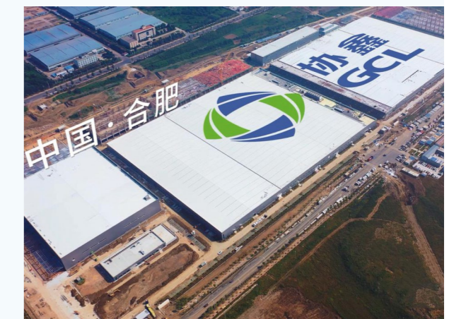
GCL S.I. (Hefei) Gigafactory
