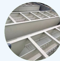
Renovation of hydrolysis tank
