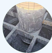
Cleaning settling tank I
